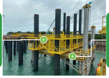
Physical protection must be installed to protect temporary works where there is a risk of collision, or damage from operating plant or live traffic.
