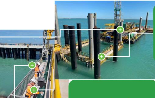
Fall Protection. All access/egress ways must be fitted with approved guardrails or other acceptable means of fall protection. Work platforms must be fully decked and guarded.
