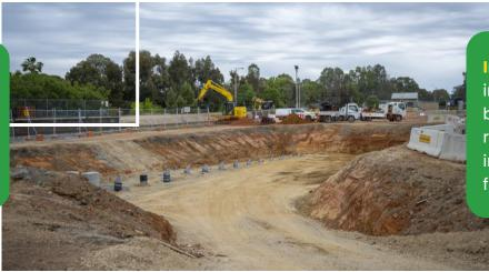
Inspection. Excavations must be inspected by a competent person before each working shift and after rainfall, or other events which could impact ground stability or introduce further hazards.
