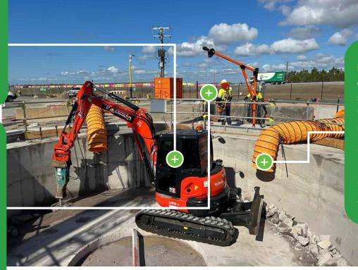
Products / Equipment used in confined spaces or potential confined spaces (e.g., trenches and open tanks) must be assessed and managed to prevent risks of:
