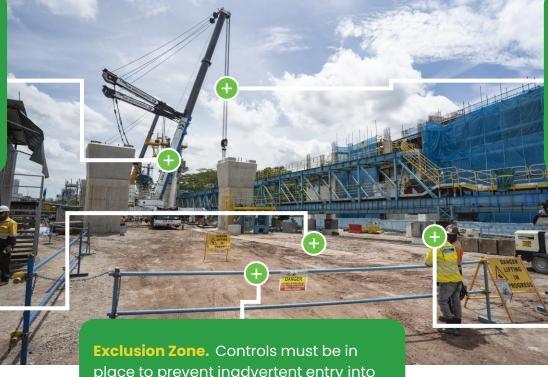
place to prevent inadvertent entry into the lifting zone. Barricades, signage or spotters shall be used as is deemed appropriate for the level of risk. Lift Plan. All Critical Lifts require a Crane Lift Plan. The Crane Lift Plan must be reviewed and verified by an Engineering Representative.
